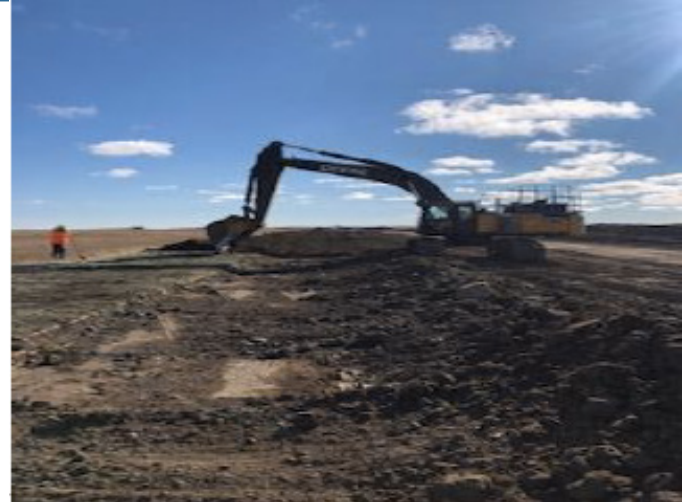
Backfill crew cleaning up spill pile – km 157+200 – Oct 10, 2018
