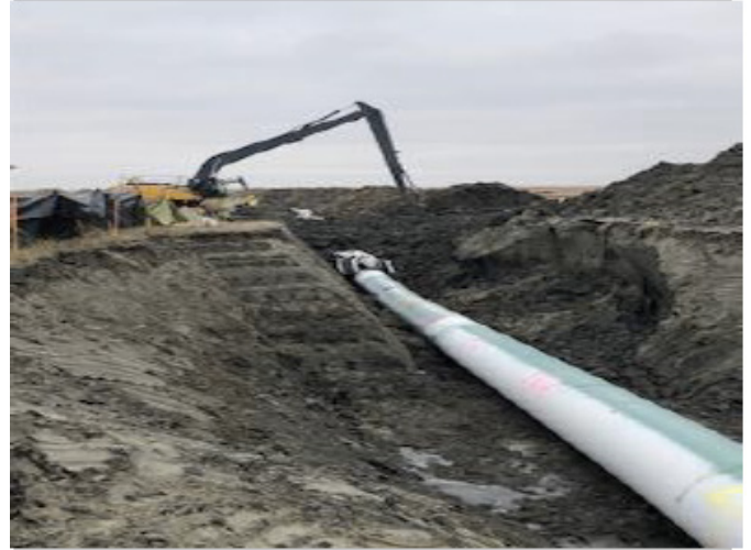
Excavators hoisting pipe weights through wetlands– SF 92 – Oct 11, 2018 Excavator shading wetland – km 152+900 - Oct 11, 2018
