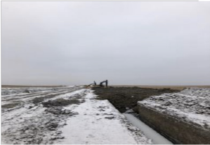
Excavator shading and cleaning – km 156+500 – Oct 9, 2018
