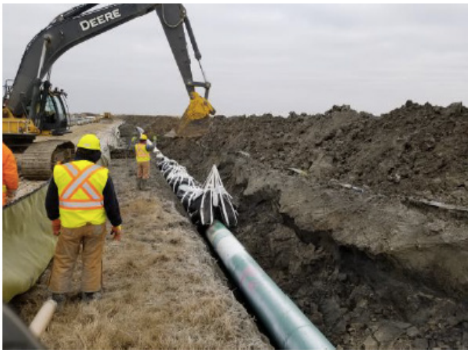
Installing pipe weights - km 152+900 – Oct 11, 2018
