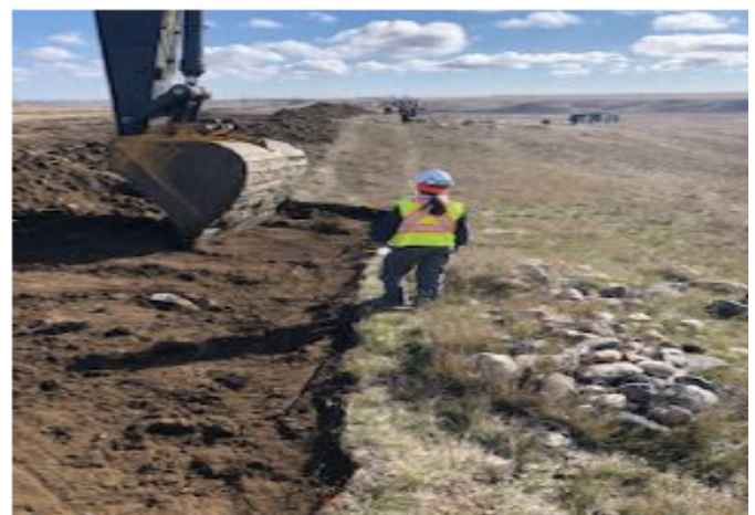
Moving topsoil back – km 153+400 – Oct 11, 2018
