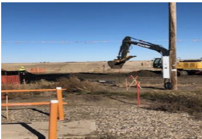
Excavator stripping ROW near power line– km 262+362– Oct 10, 2018
