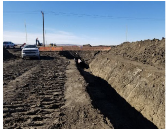
Pulled bore –km 233+247– Oct 10, 2018
