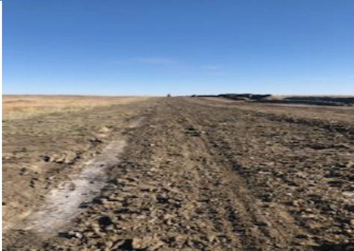
Backfilled mainline – km 154+600 – Oct 10, 2018
