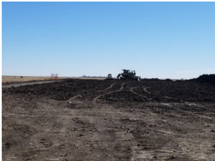
Equipment moving dirt – km 257+525 - Oct 10, 2018
