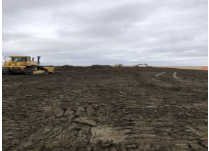
Transition soil being piled– km 259+680 – Oct 9, 2018
