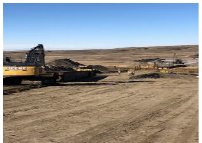
Bridge being moved to watercourse– SF 162 – Oct 10, 2018
