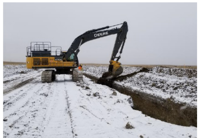
Transition soil being piled– km 259+680 – Oct 9, 2018
